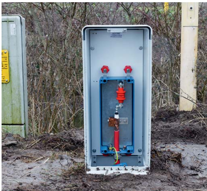
Coaxial connection of the Ex isolating spark gap for protecting buried insulating joints
