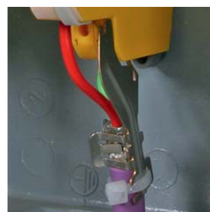
EMC spring terminal for permanent low-impedance shield contact.
