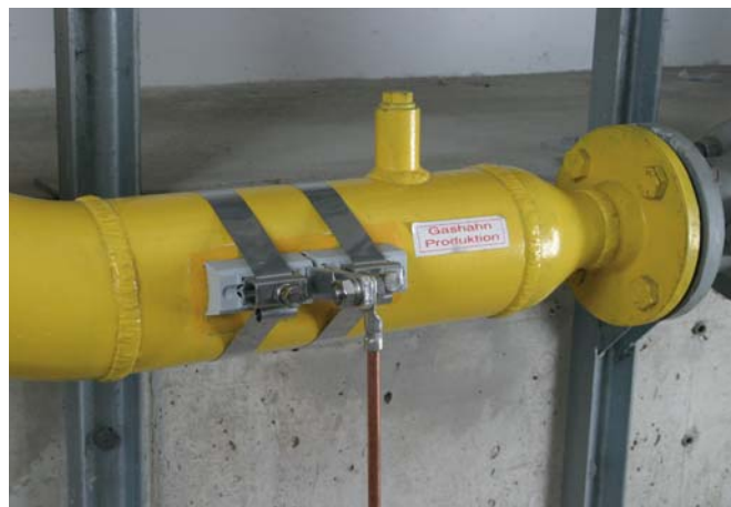
Pipe clamp for electrical contacting of pipes in explosion-hazardous areas for implementing of lightning equipotential bonding according to IEC/EN 62305-3
