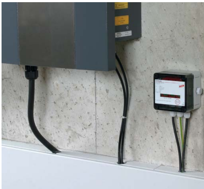
For protecting low-voltage consumer's installations against surges. For use in accordance with IEC 60364-7-712 (installation of photovoltaic power supply systems).
